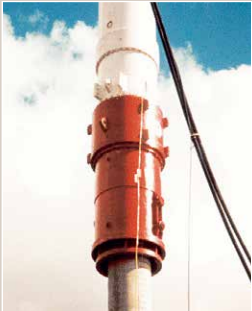
SC-hammer driving freehanging spun piles
